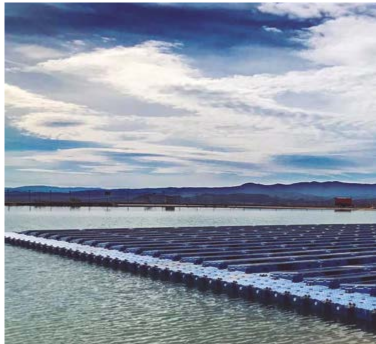
Floating solar pumping on raft and two underground pumps for self-consumption in the Irrigation Community of Llíria, Valencia (Spain)
